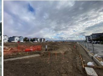
Construction of the two-acre Forest Park along Central Parkway, Pino Grande Road, Twain Harte Road, and Pandora Way is underway. The contractor is currently working on underground utilities, perimeter sidewalks and interior pathways, as well as paving the multi-use, asphalt sports court.
