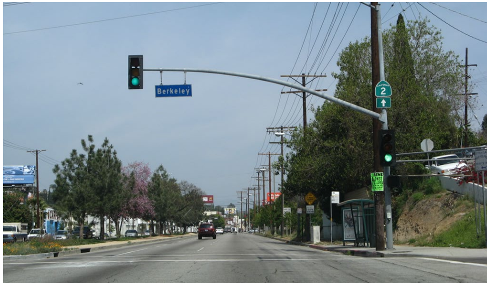
Figure 5. Example of Mast Arm
