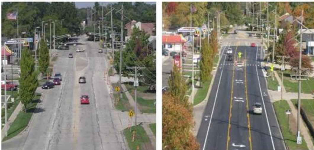
Figure 32. Example of Road-Diet (Roadway Cross-Section Before and After Reconfiguration)
