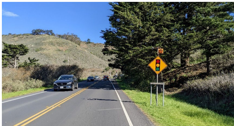
Figure 12. Example of Flashing Beacons as Advance Warning
