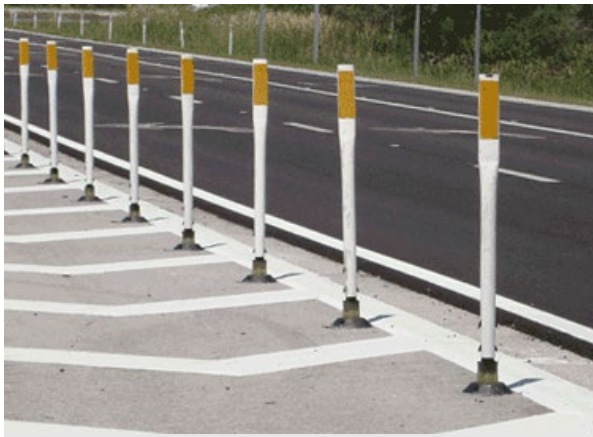
Figure 39. Example of Roadside Delineators
