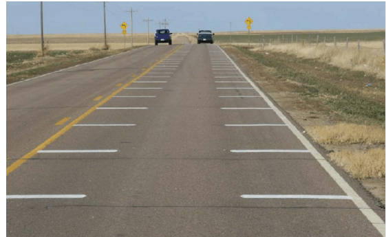
Figure 29. Example of Optical Speed Bars
