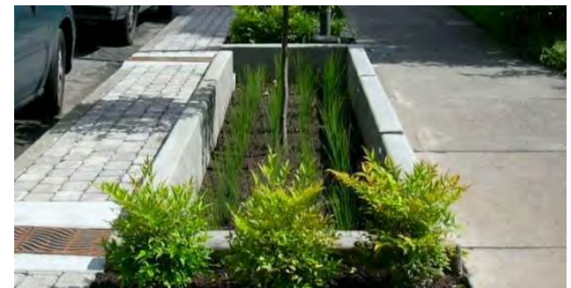
Example of a flow through planter
