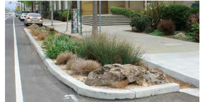
Example of a bulb-out used to capture stormwater runoff
