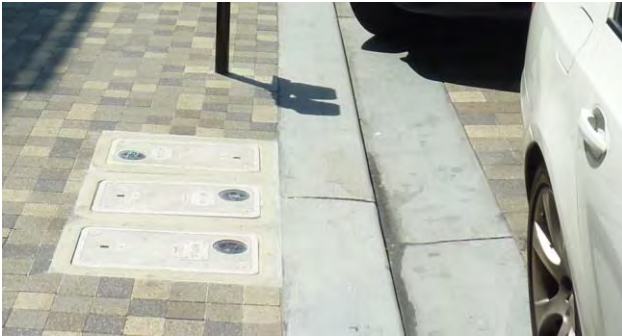
Example of utility boxes grouped together to reduce visual clutter in the sidewalk
