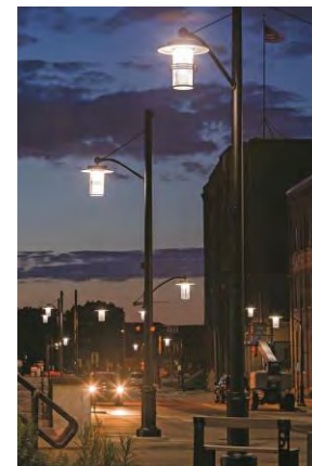
Example of roadway lighting with pedestrian lighting on the back of pole
