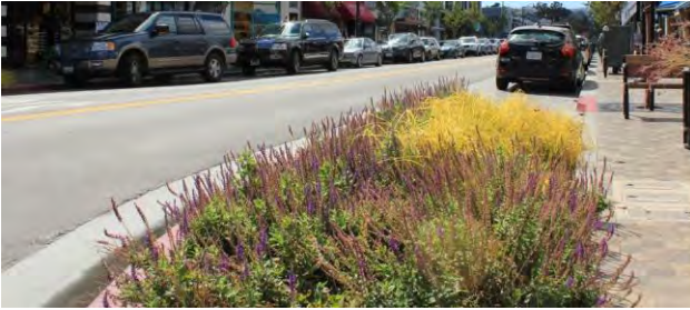
Stormwater planters at bulb-outs capture runoff before entering the storm drain system
