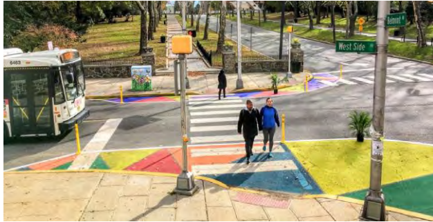
Paint used to extend pedestrian safe space beyond the curb to reduce crossing length
