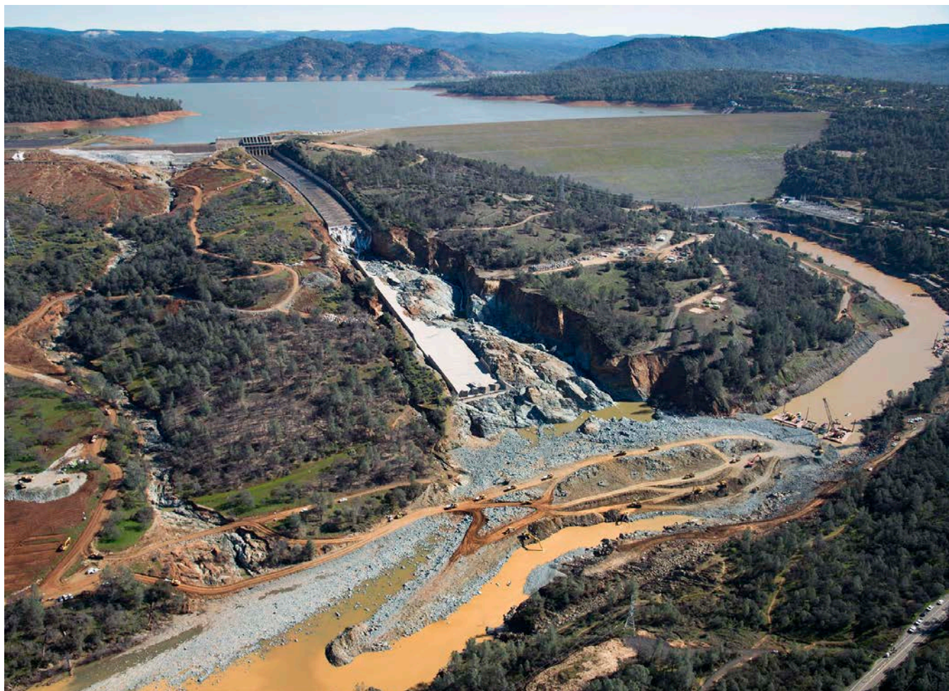
Figure 13-5. Oroville Dam Emergency Spillway Failure in Spring 2017
